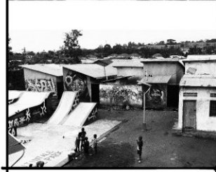
EXISTING SKATE RAMP WITH BACK-DROP OF HOUSES
