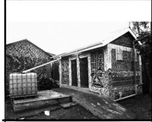
EXISTING WATERBORNE TOILET (note that the watertable is high)
